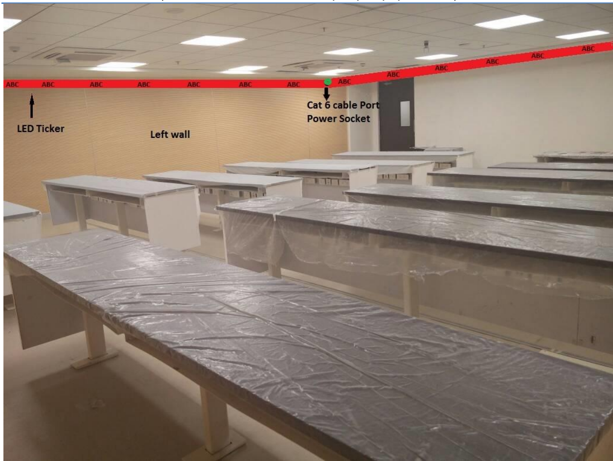
Picture 3: location of RJ45 port and power socket on the ticker display
